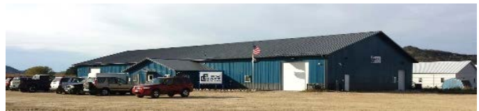
Pictured above – Flex Craft's Houston, MN Manufacturing Facility
